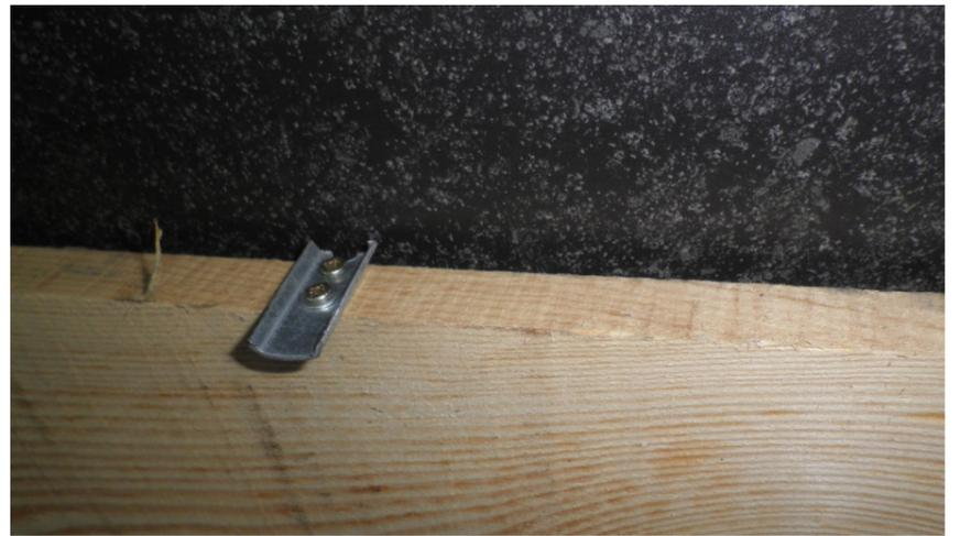
3. Place the plank in between the slab(s) you want to lift. Make sure the plank is placed on the backside of the slab, where the fiberglass mesh is glued.
