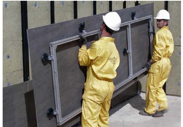
Image 7: Slab handling with Suction Frame
