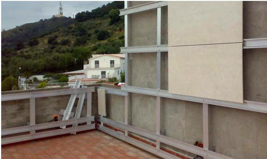
Image 50: Strongfix System installation Step 2 and 3
